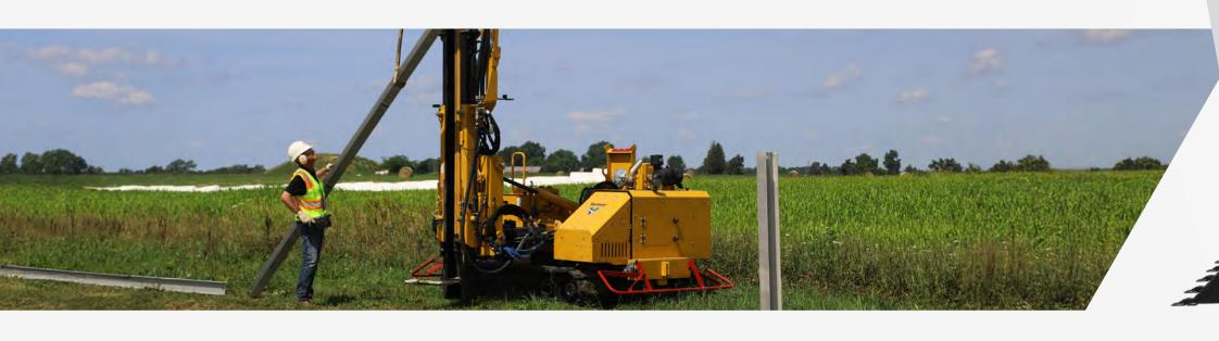
Constructing the actual solar panels is a multi-step process: First, the piles need to be laid and driven into the ground. Second, the racking needs to be assembled to the piles. And finally, the solar panels can be installed on the racking. Precision and efficiency are extremely important in the equipment installation phase, and Vermeer installation equipment meets the challenges of these jobsites.
